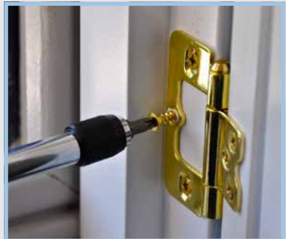
Final fix of 3rd screw in shutter hinge.
