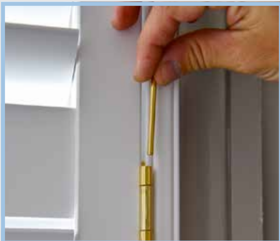
2 parts of hinge coming together with drop pin going in.
